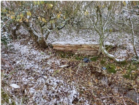
Figure 2.3 Inlet pipe (looking downstream at SP 52927 26132)
