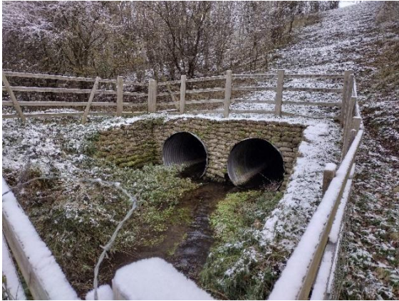
Figure 2.28 Twin culvert under M40 motorway (looking downstream at SP 54607 28232)
