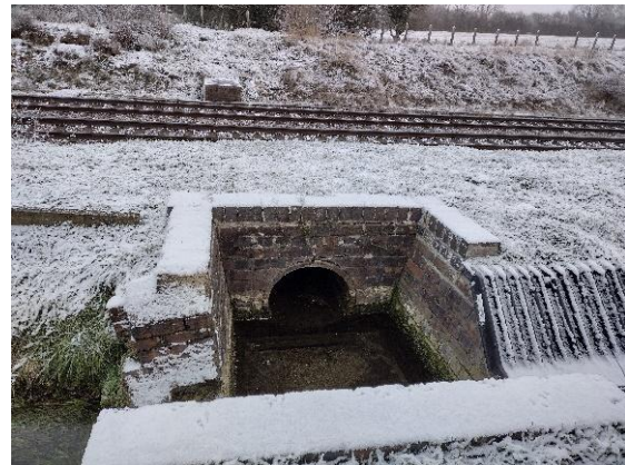
Figure 2.25 Culvert under railway (looking downstream at SP 53131 27573)
