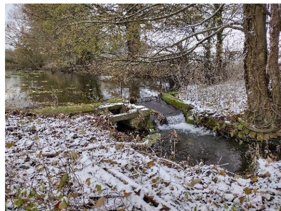
Figure 2.14 Online pond and downstream weir (looking upstream at SP 53131 24639)
